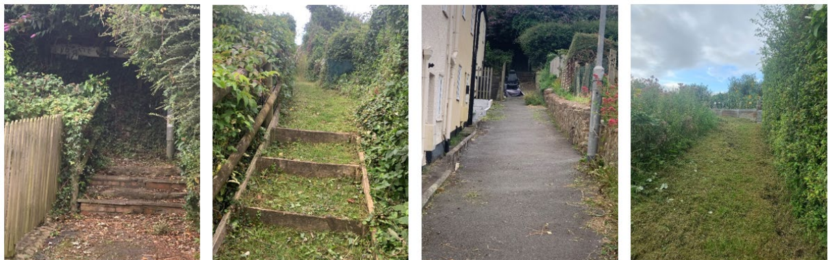
Image 8.2 – Public footpath conditions (narrow widths, steep gradients and steps)
